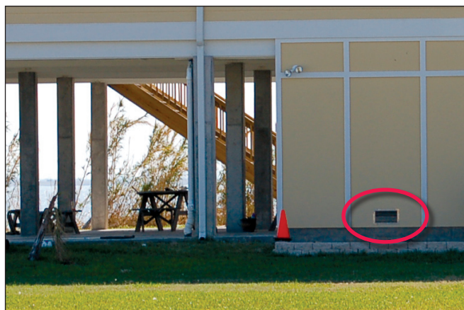
Figure 5. Flood opening in a below-BFE enclosure wall.
