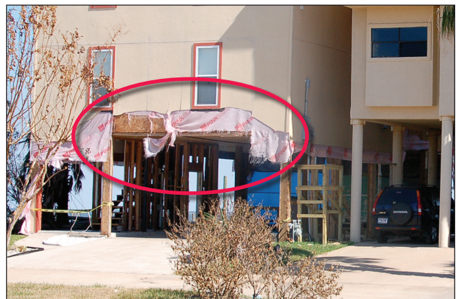
Figure 3. NFIP-compliant breakaway wall construction.
